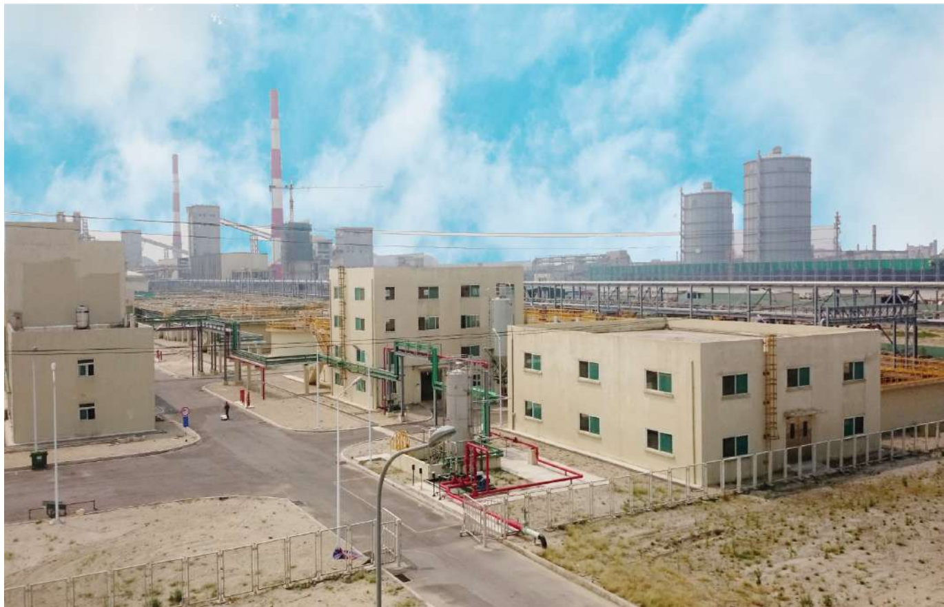
Formosa Wastewater Biological Treatment Plant
